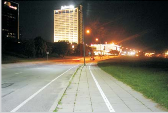
LED Street Lighting
